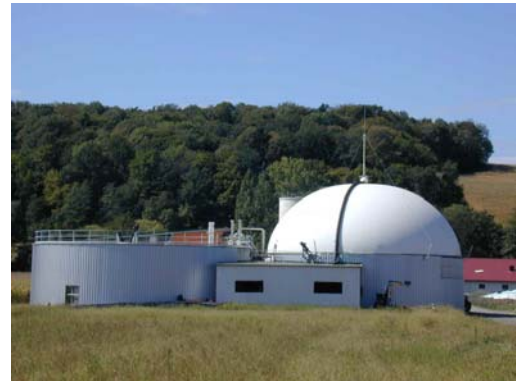
Biogas Plant St. Stefan © Rosentaler Bio Power
