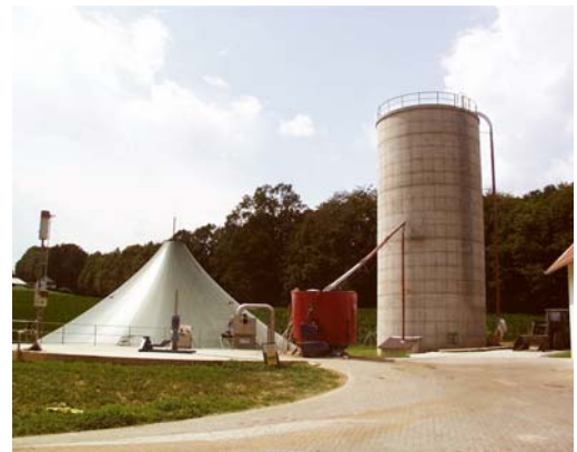
Biogas Plant St. Georgen © LEA
