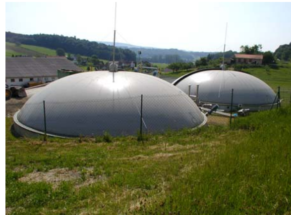
Biogas Plant Ebersdorf © LEA
