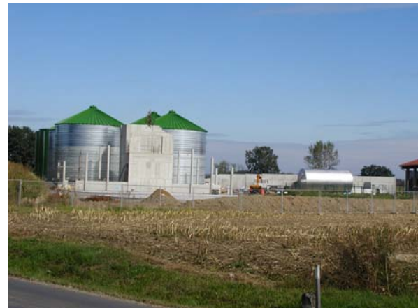
Biogas Plant Mureck © LEA
