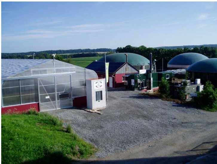
Biogas plant Thomas Karle © Karle
