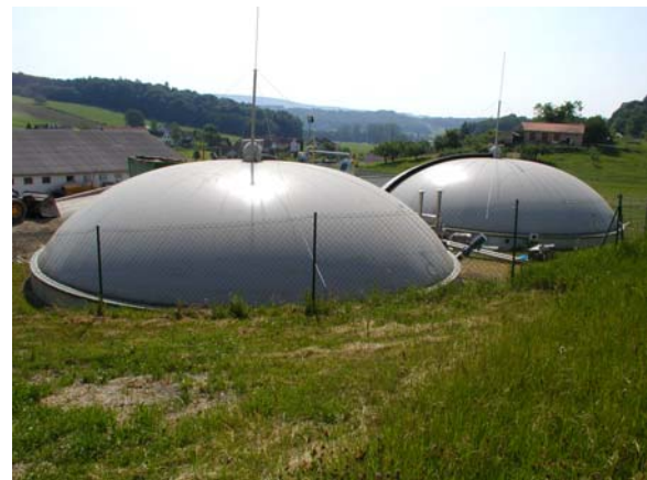
Biogas Plant Ebersdorf © LEA
